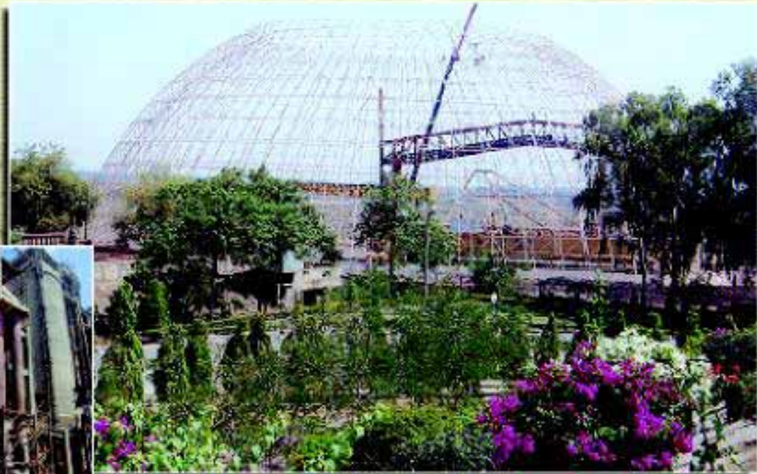
The specially designed Circular Stacker Reclaimer Dome shed (first such facility in India) and (inset) the new Vertical Pregrinder Raw Mill at Satna
