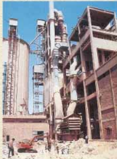
Excavation work for the CCW Raw Grinding Vertical Roller Mill
