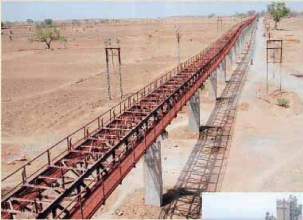
The 3.97-km-long cross-country 1,200 TPH Belt Conveyor, under installation, for carrying limestone from the quarry to the new circular stacker yard at Satna
