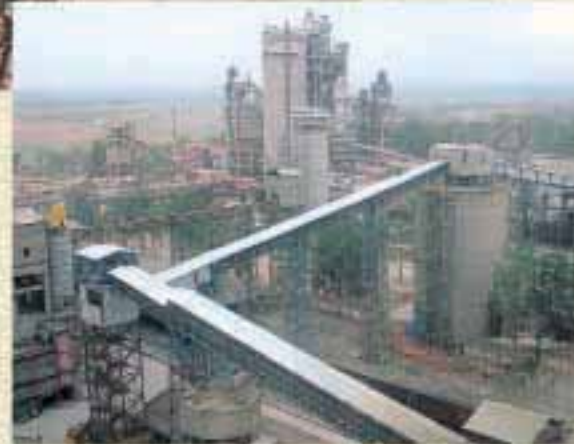
The clinker silo and wagon-loading facility at Satna
