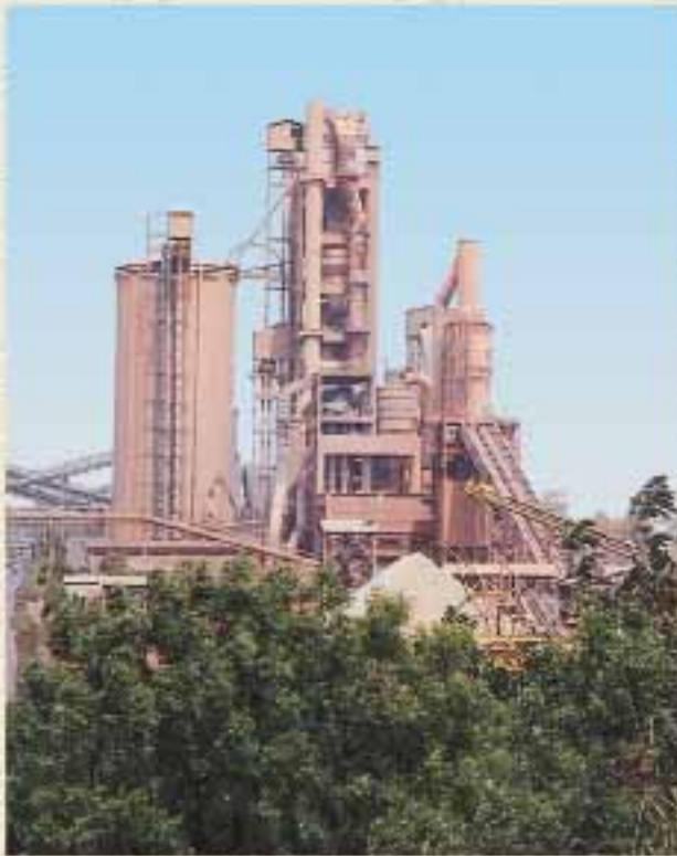
An overview of the CCW plant with the newly installed CF Silo Feed Bucket Elevator on the left
