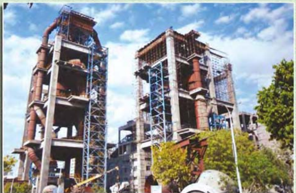
The first and second roller press buildings at the upgraded Chanderia Cement Works, Chanderia.
