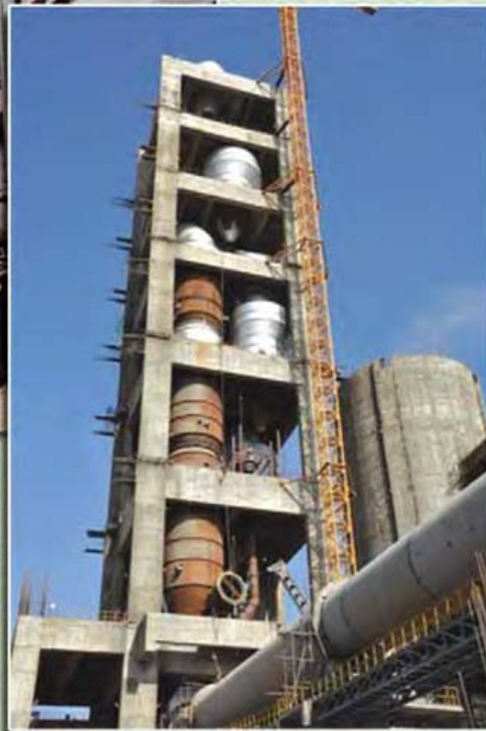
The preheater tower at Birla Vikas Cement, Satna (top) and the preheater tower of New Chanderia Cement Works, Chanderia (right).
