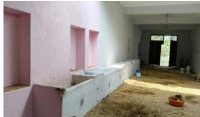
Construction of manger for animals
