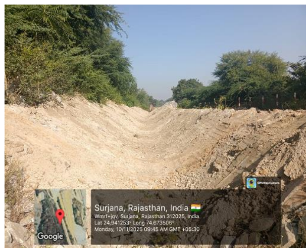
Garland drains structures are constructed around the over burden dumps
