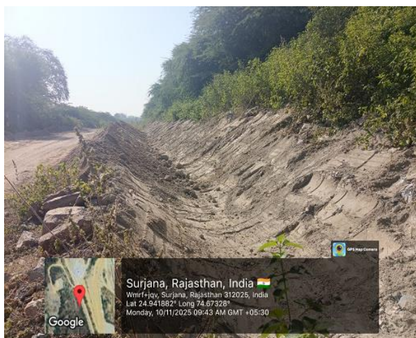
Garland drains structures are constructed around the over burden dumps
