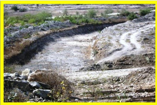
Garland Drain Along Dumps
