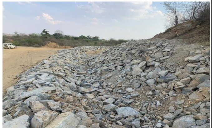
Garland drains structures are constructed around the over burden dumps
