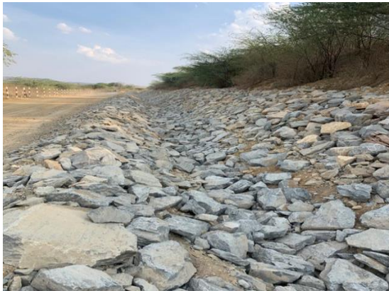
Garland drains structures are constructed around the over burden dumps
