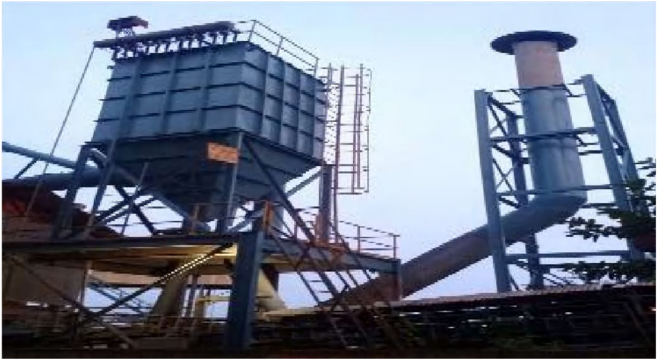
Bag Filter installed at transfer points
