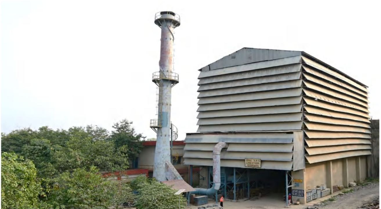
Bag House installed at covered Crusher
