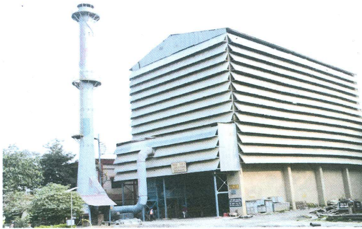
Fully Covered Crusher House with Bag Dust Collector
