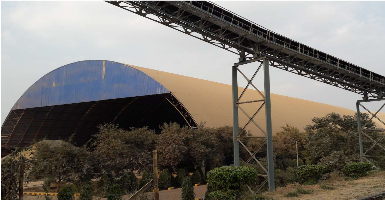
Linear Limestone Storage Yard- BVC Plant
